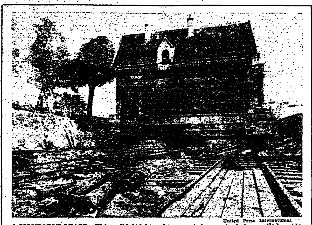
A MOVEABLE LEASE —This solid brick and cement house is being rolled aside some 50 yards to make room for new circular expressway being built around Paris. But it will not be destroyed and once the work is done, will again be a home.
